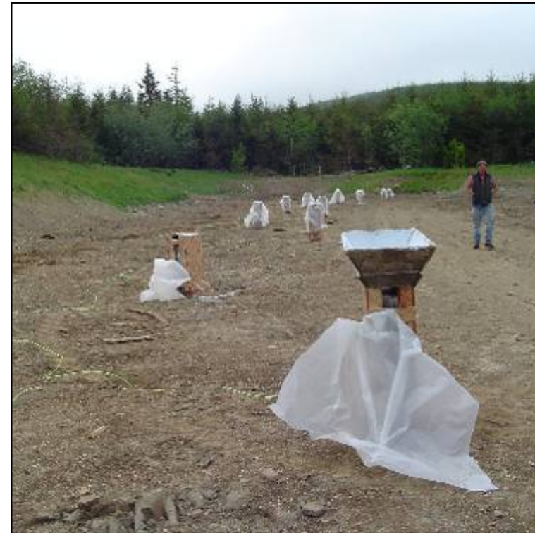
Hoppers for pouring explosives into charge gap
