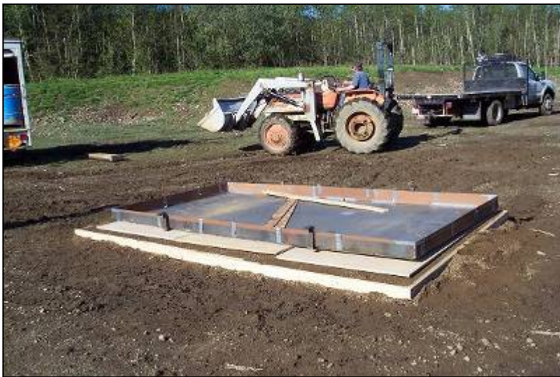
Final shot readied for detonation
